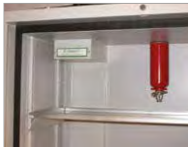
Fire-extinguisher installed in a safety cabinet
